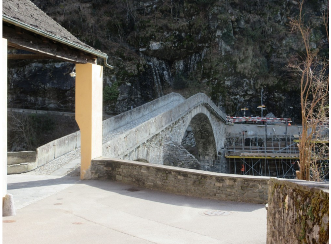
Steinbrücke in Bignasco
